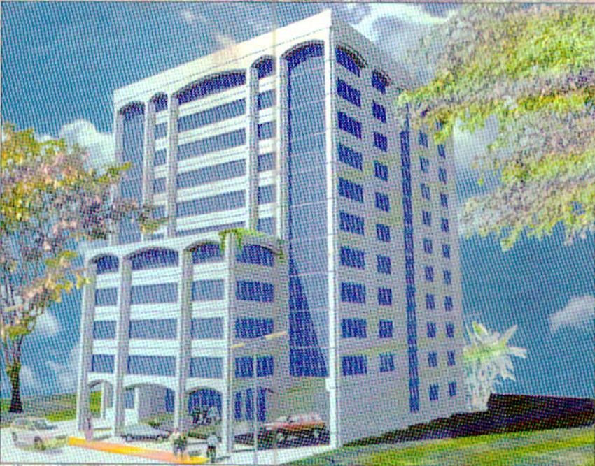
Judicial Administration Training Institute Complex (under construction).
